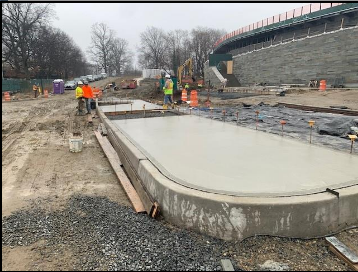
Sidewalk Paving and Site Lighting Pole Installations
