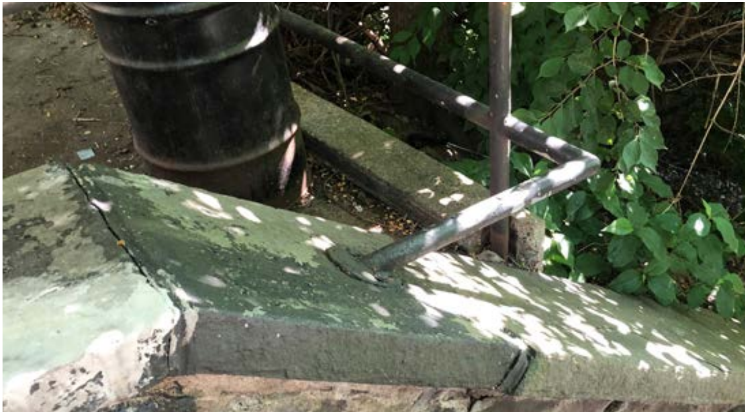
1 - Looking at entry cheekwall and sidewalk railing and curb wall
