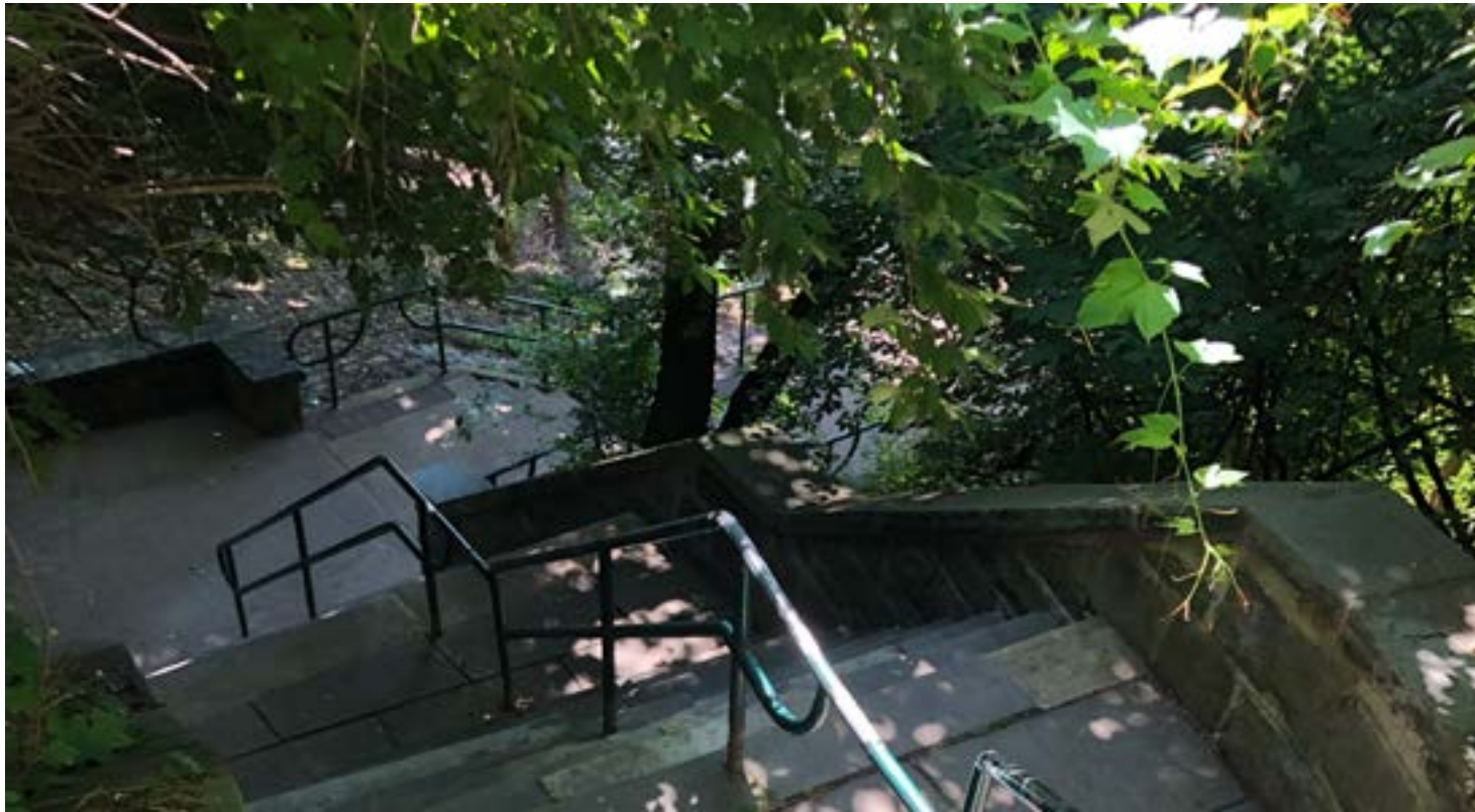
1 - Looking down stair
