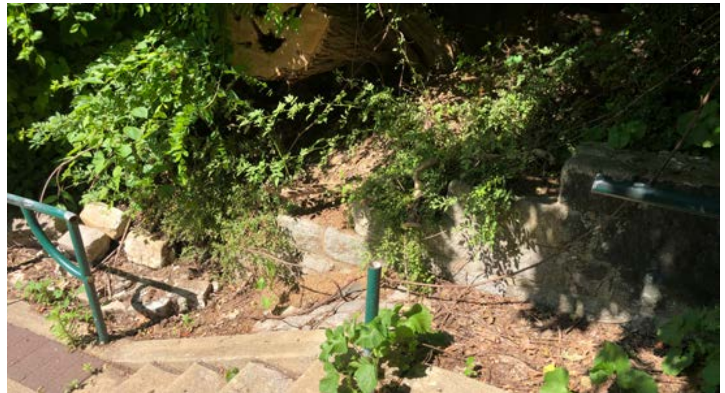
2 - Retaining wall at slope base
