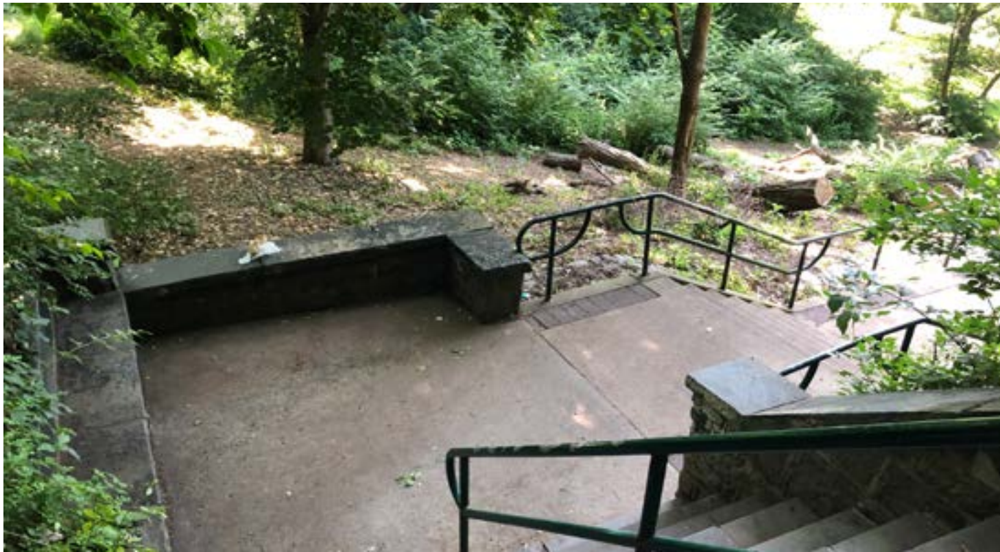
1 - Looking down at bottom landing entry
