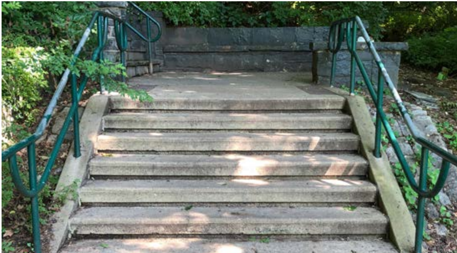
1 - Looking at lower entry landing at stepped walkway
