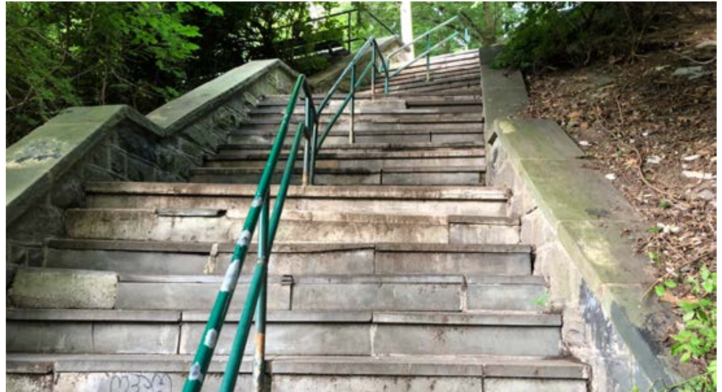
2 - Looking up stairway
