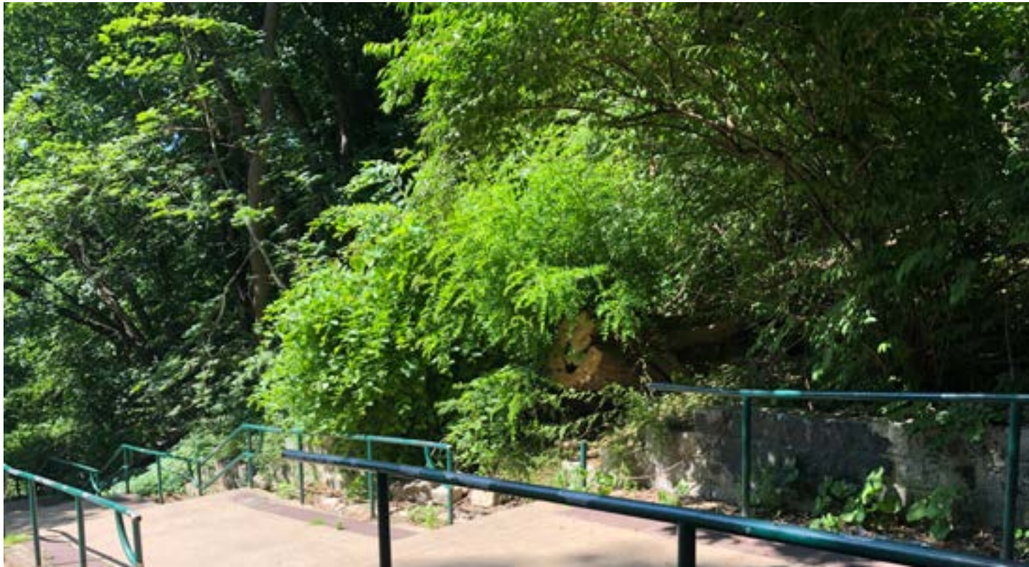
1 - Looking southwest at slope along stepped walkway
