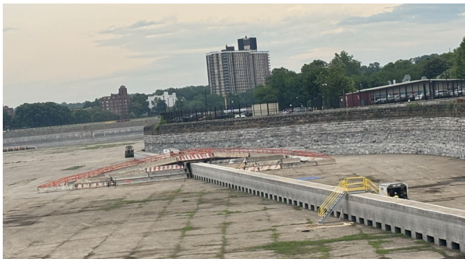
Temporary Ramp and Walkway South Basin
