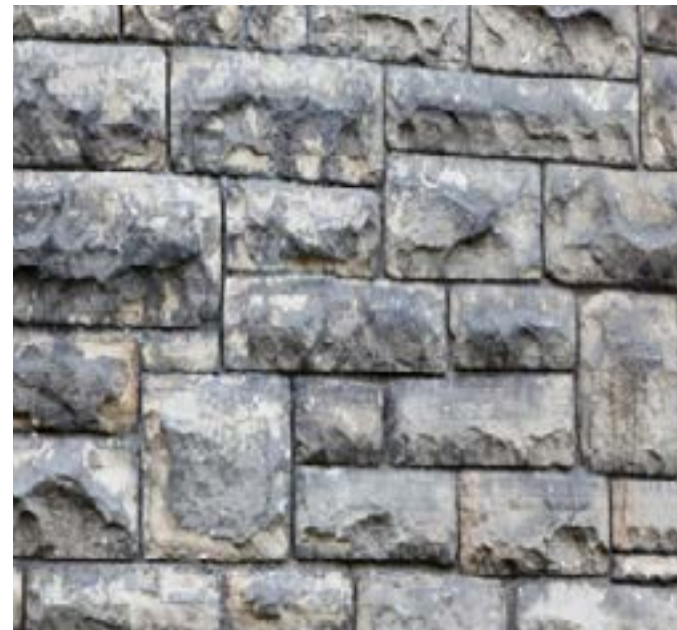
GNEISS VENEER WALLS, MATCH EXISTING
