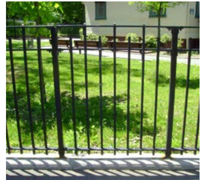
3'-6" HT. STEEL BAR FENCE
