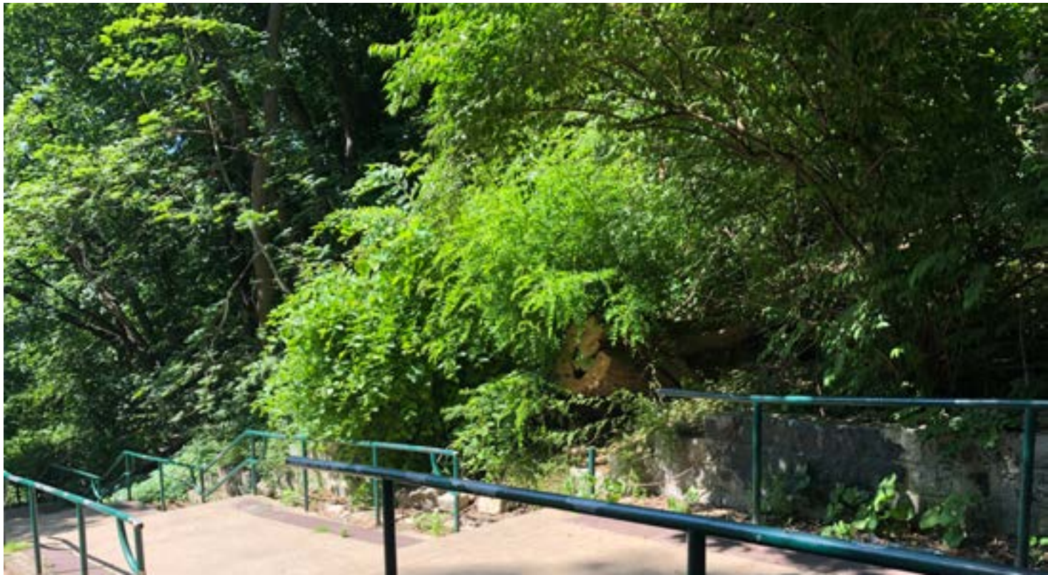
1 - Looking southwest at slope along stepped walkway
