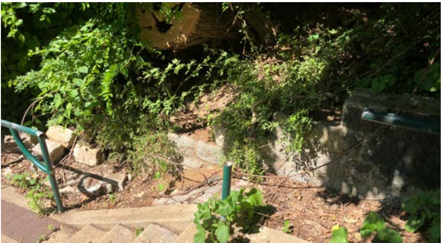
2 - Retaining wall at slope base
