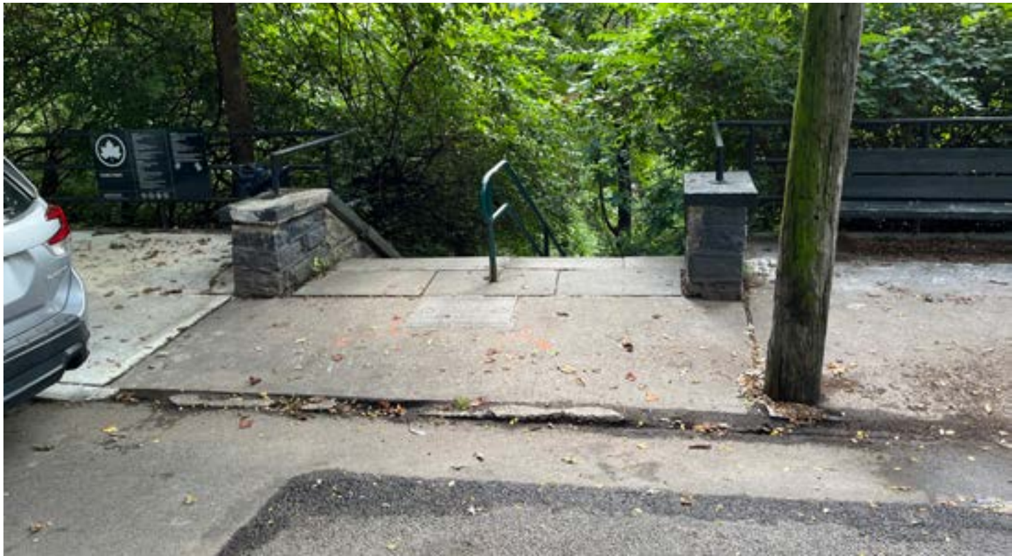
1 - Johnson Ave. Entry
