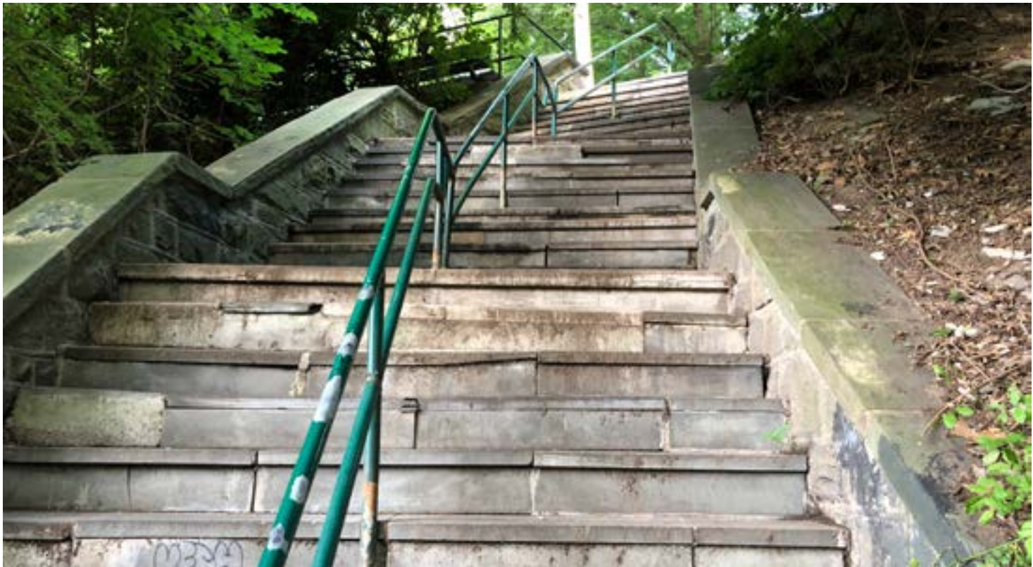
2 - Looking up stairway
