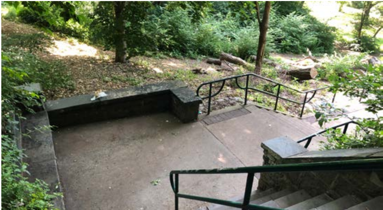
1 - Looking down at bottom landing entry
