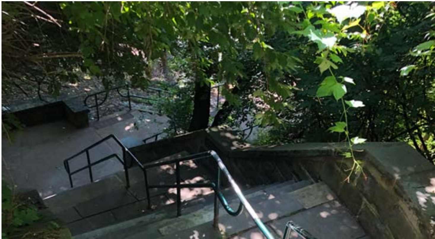
1 - Looking down stair
