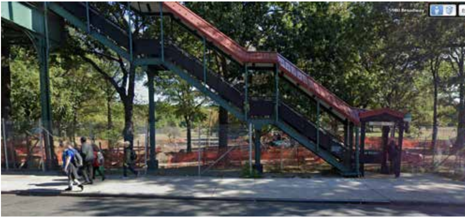
Figure 36- Space under 242 Street stairway, east side of Broadway
