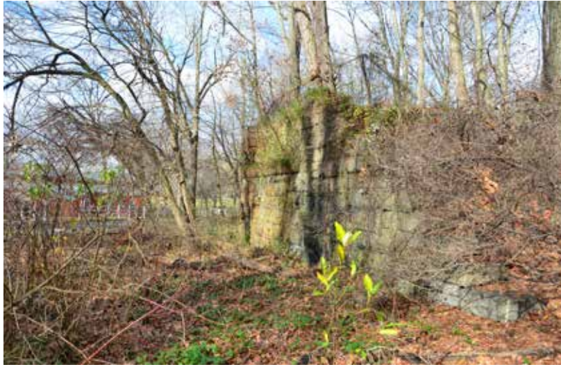
Figure 29- area of proposed pedestrian bridge over old abutment
