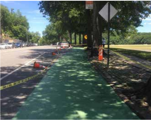
Figure 32 - Bike lane under construction
