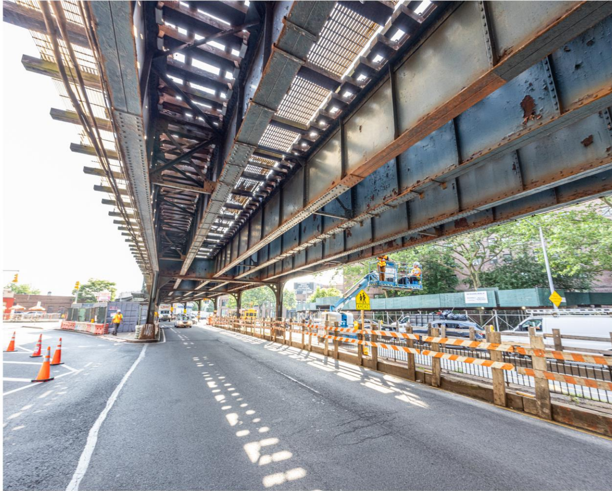
EL SOL CONTRACTING/ES II ENTERPRISES JV MTA C&D CONTRACT NO. C35328 PAINTING AND STEEL REPAIRS OF ELEVATED STRUCTURES: 225TH STREET TO 242ND STREET ON THE BROADWAY 7TH AVE. LINE (IRT) IN THE BOROUGH OF THE BRONX VIEW: BENT 175W > NE PHOTO: 14266.003.006 DATE: 06/12/2025 08:41AM
