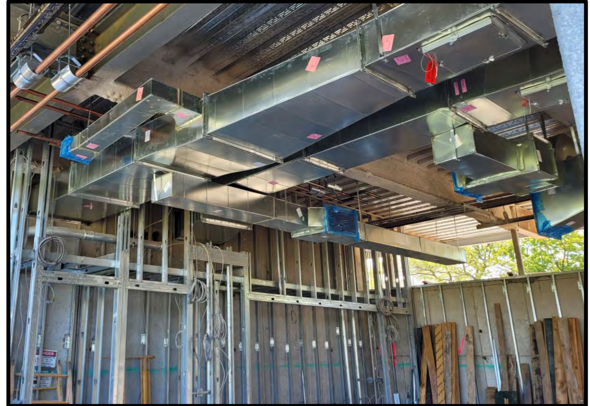
First Floor Ductwork
