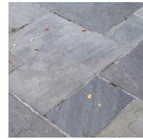
4" thick bluestone slabs
