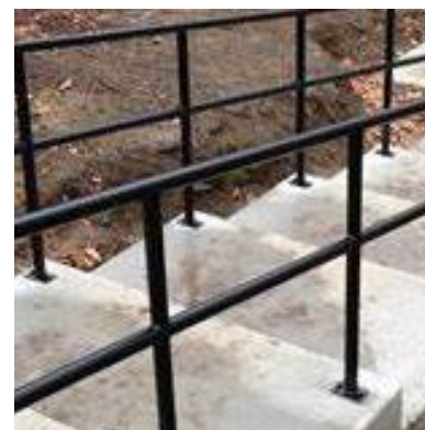
Painted steel railing
