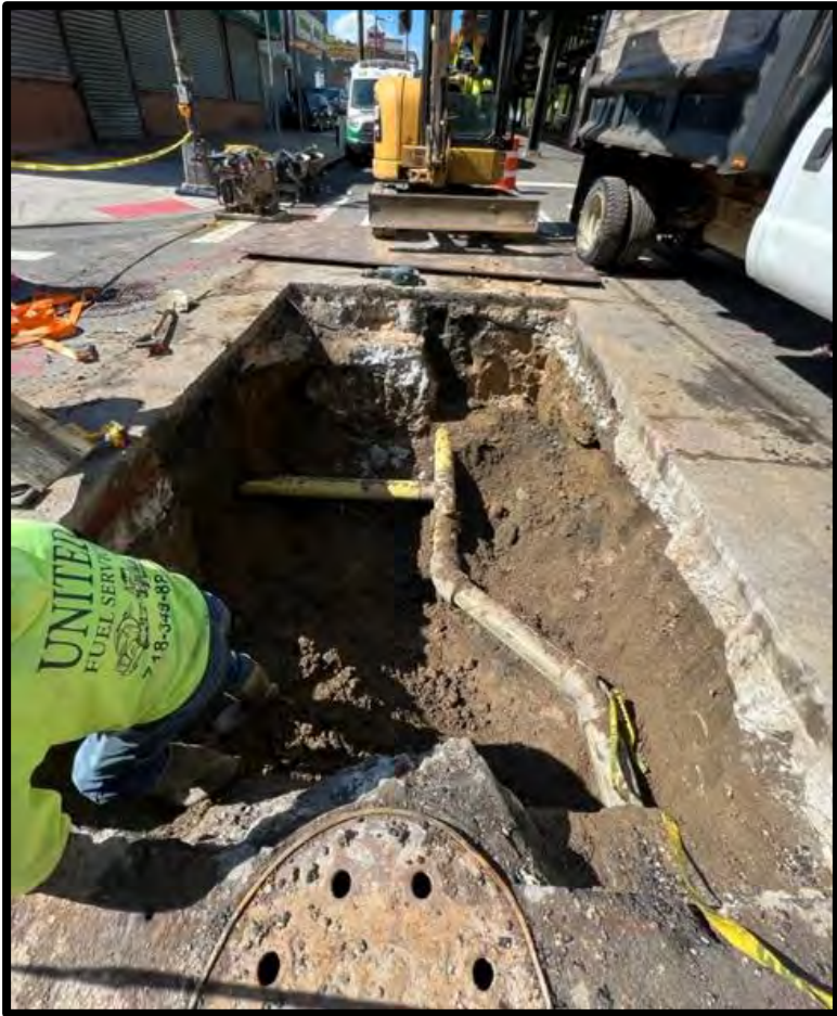
Water/Sewer Test Pit
