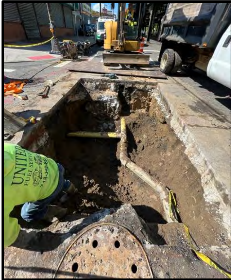
Water/Sewer Test Pit
