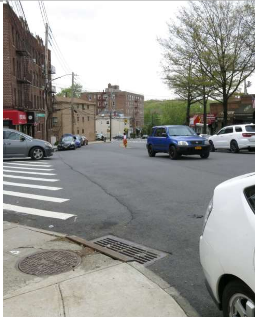
Mosholu Avenue approaching Tyndall Avenue
