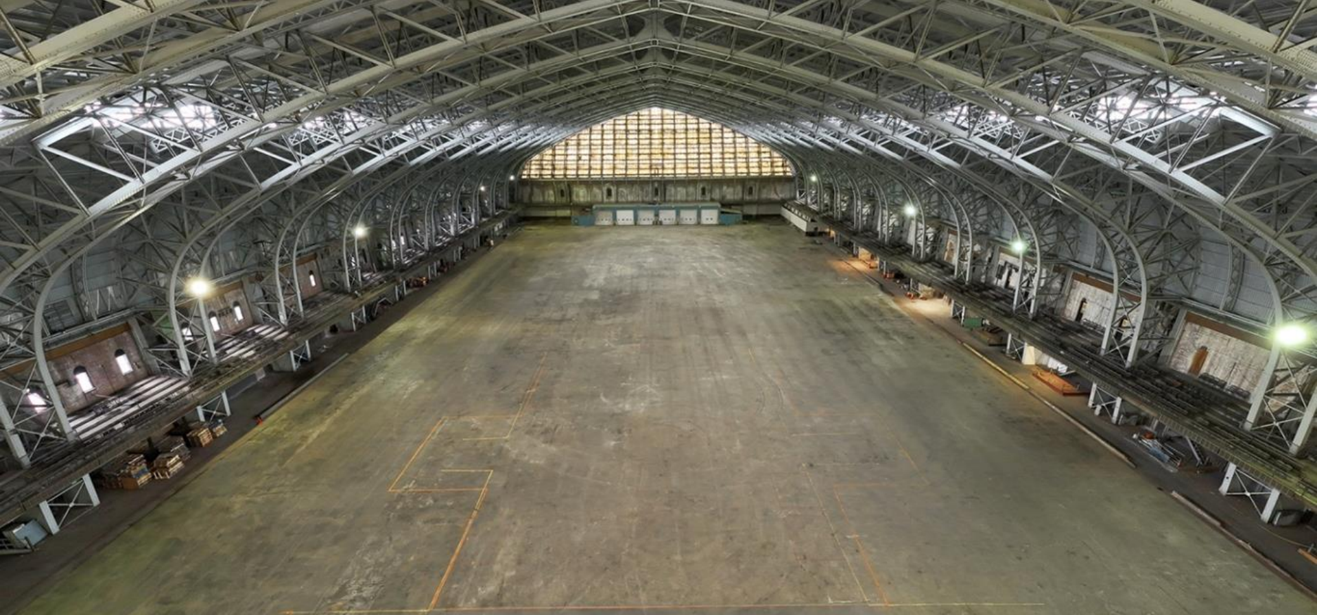
The drill hall is 180,000 SF and 115' tall at its highest point
