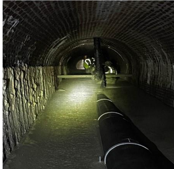
DIVERSION PIPE, BULKHEAD AND CLSM PLACEMENT WITHIN OLD CROTON AQUEDUCT BETWEEN GATEHOUSE 5 AND GATEHOUSE 7
