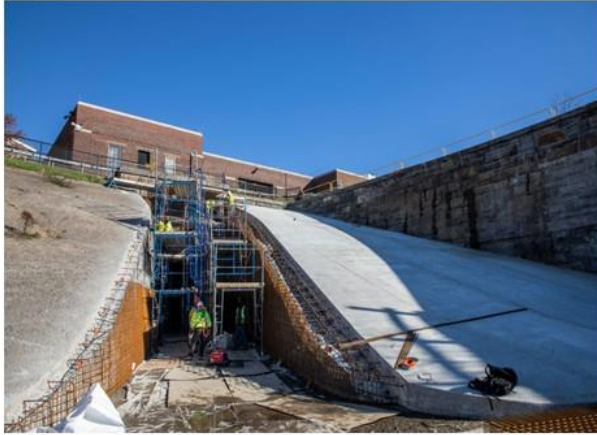
NORTH BASIN INLET SHOTCRETE AND EMBANKMENT SLAB REHABILITATION
