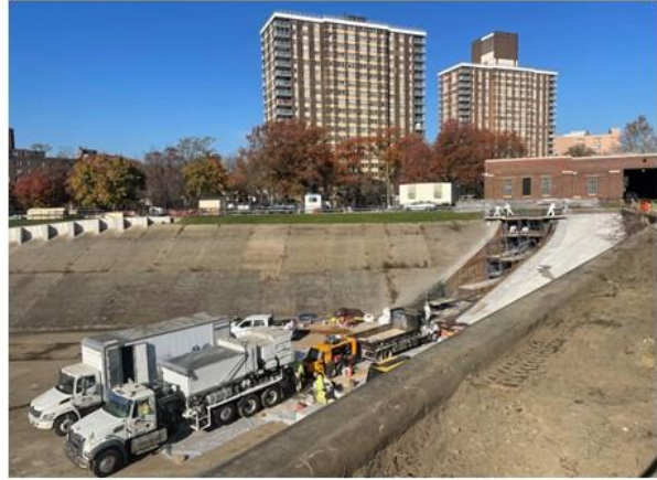
NORTH BASIN INLET SHOTCRETE AND EMBANKMENT SLAB REHABILITATION
