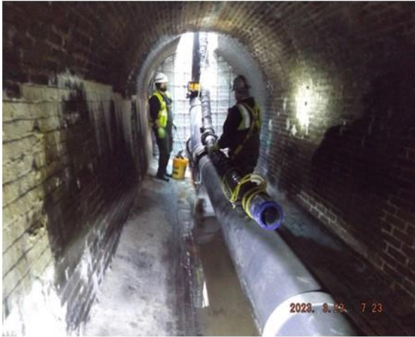
DIVERSION PIPE, BULKHEAD AND CLSM PLACEMENT WITHIN OLD CROTON AQUEDUCT BETWEEN GATEHOUSE 5 AND GATEHOUSE 7
