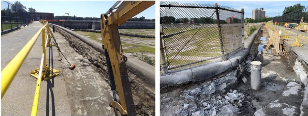
EAST ROADWAY GRADE BEAM EXCAVATION AND SHEETING
