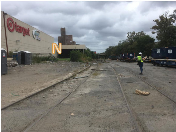
07 View of the MTA Metro-North Right-Of-Way and the adjacent parcel to the west facing northeast
