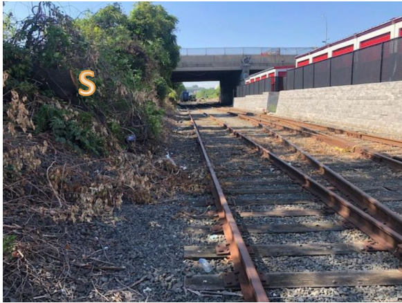
05 View of the MTA Metro-North Right-Of-Way and the adjacent property to the west facing south
