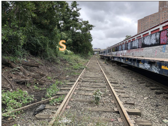
03 View of the MTA Metro-North Right-Of-Way facing south
