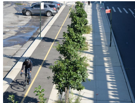
Raised Bike Lane
