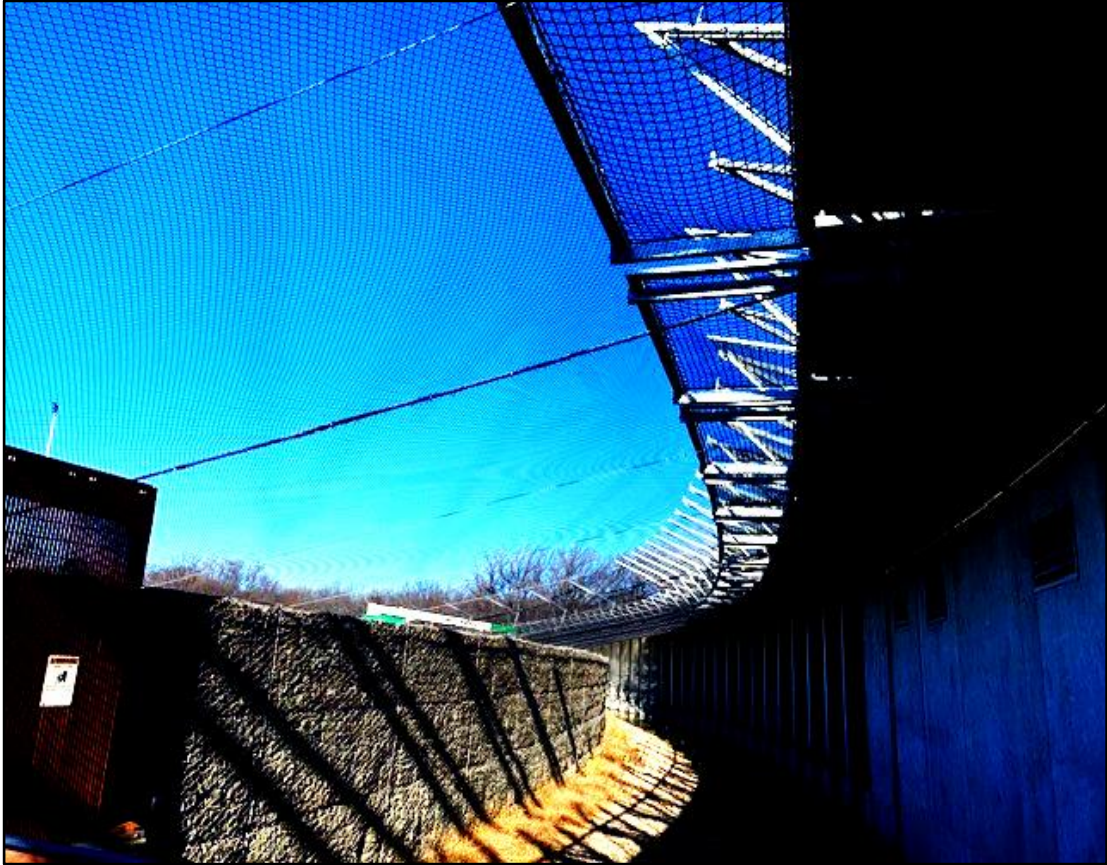
Ball Collection Netting Installation
