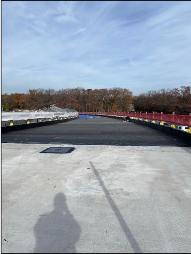
Waterproofing on Roofing
