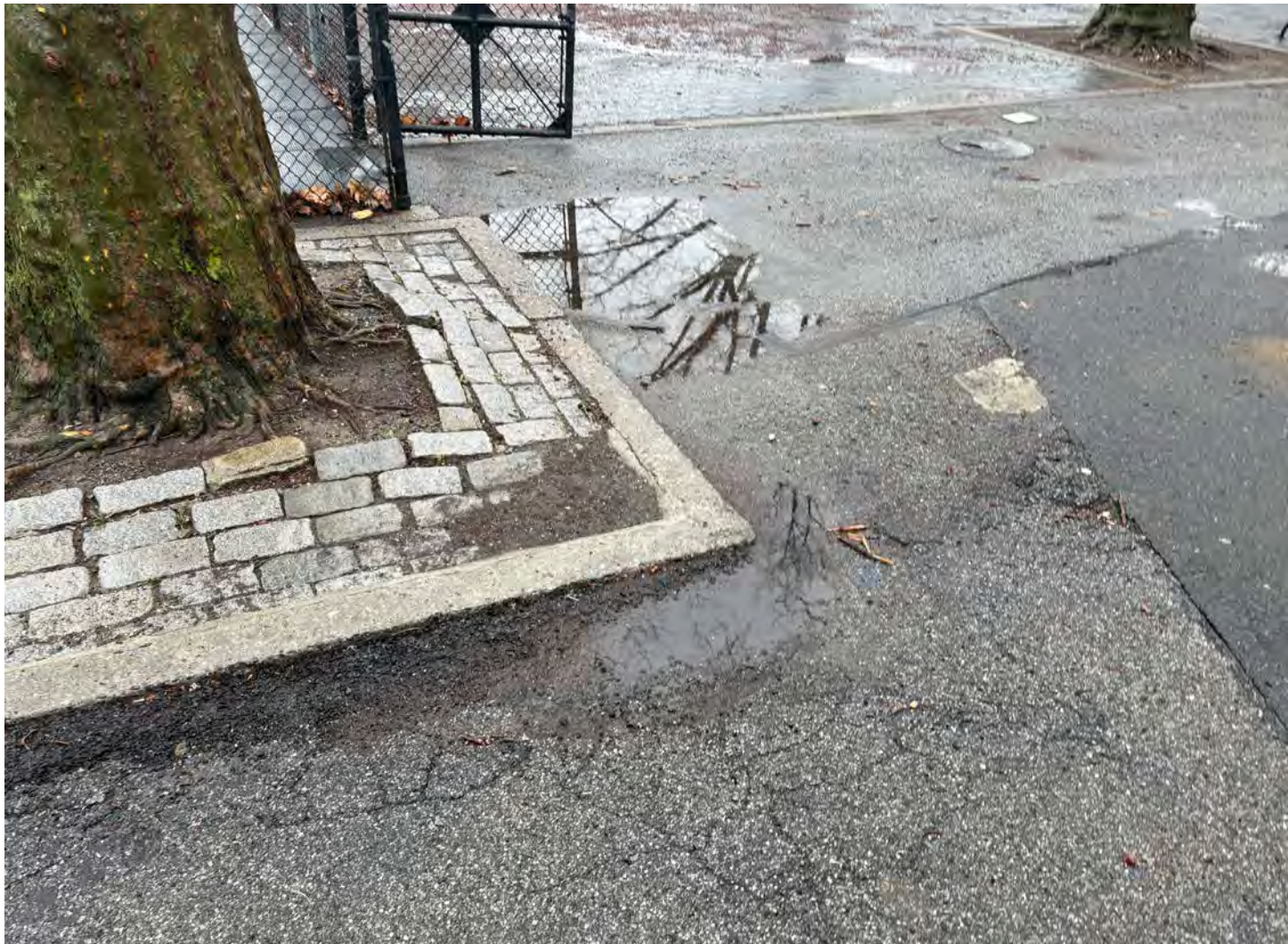
5 - Tree pit with granite block
