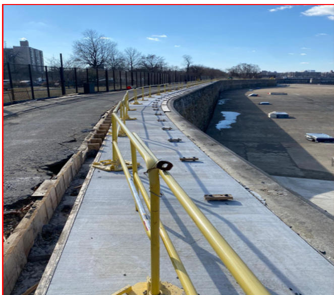
Construction of the Grade Beam Along East Road
