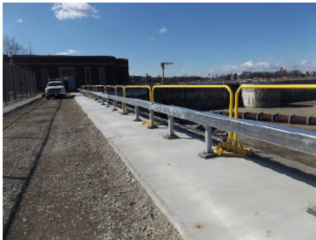
Construction of the Guide Rail Along the East Road
