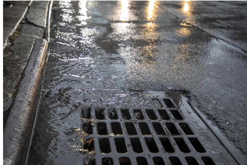
Cleared Catch Basin
