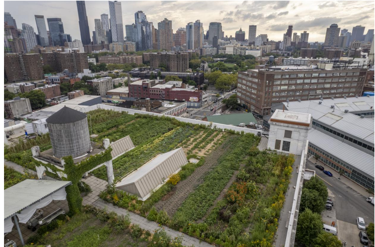
Green Roofs Absorb Stormwater
