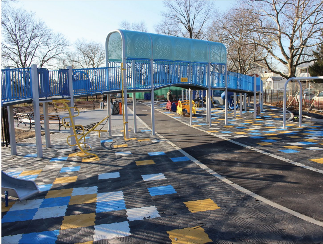
Laurelton West Playground - Full Ramping
