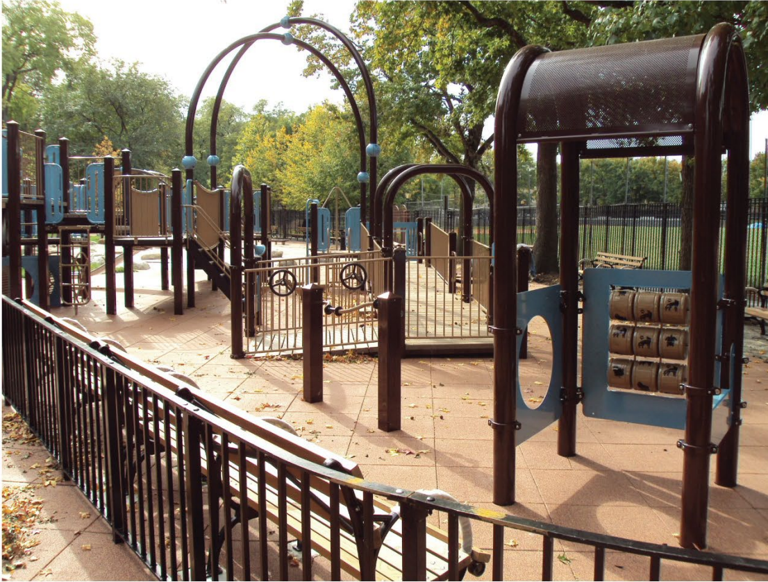
Indian Road Playground - Partial Ramping
