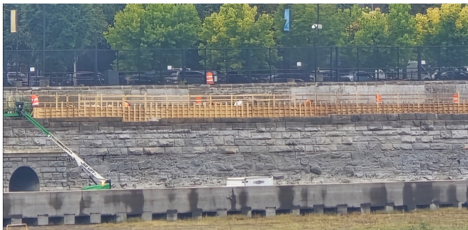
Formwork for South Road Grade Beam
