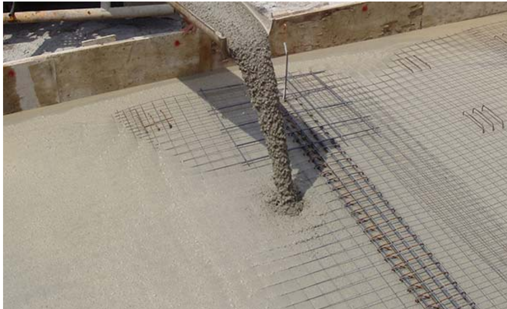
Flowable, self-leveling concrete (image: www.chaneyenterprises.com )
