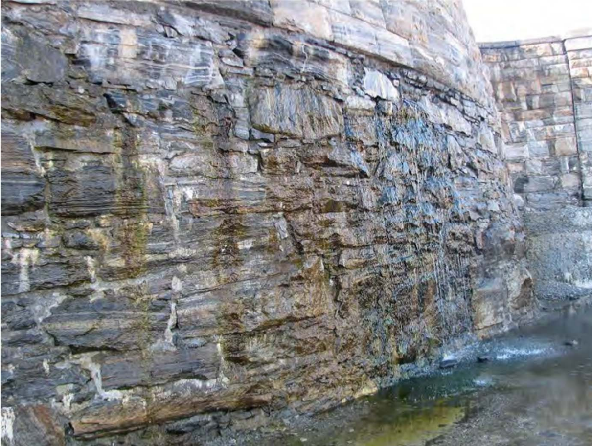
Leakage into the reservoir basin and deterioration of the east wall
