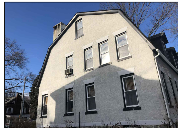
VIEW OF SOUTH ELEVATION
